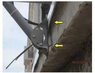
Current satellite dish installation is improperly installed and unsecure.
