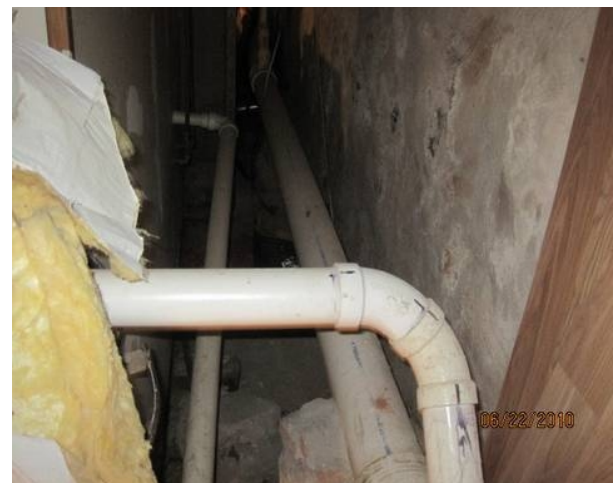
Drain pipes in the basement are satisfactory.
