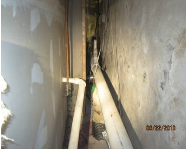
Drain pipes in the basement are satisfactory.
