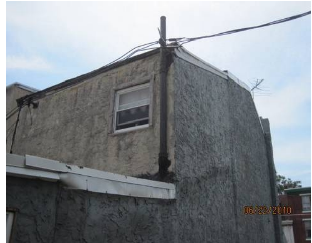
Long view of the vent stack.
