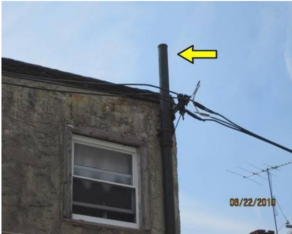
The satellite dish was reported to have been removed from the rear stack vent by the satellite company.
