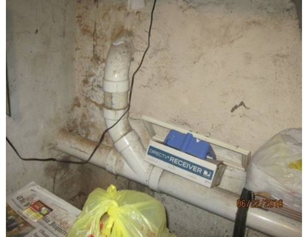
Drain pipes in the basement are satisfactory.
