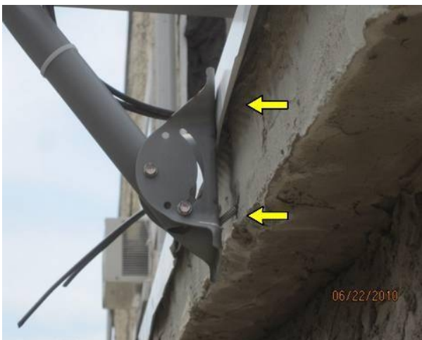
Current satellite dish installation is improperly installed and unsecure.
