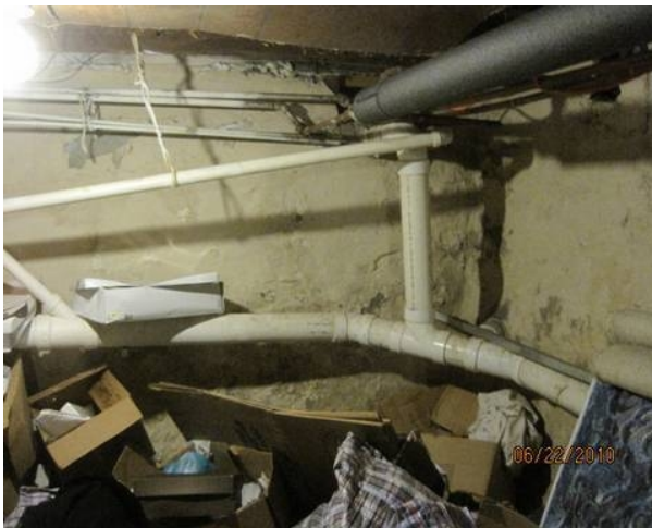
Drain pipes in the basement are satisfactory.
